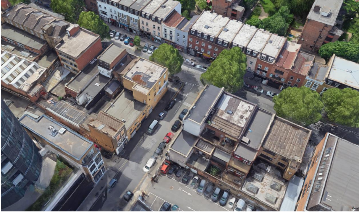
Fig 3: Aerial view of the site from the northeast looking towards the junction of Fonthill Road and Goodwin Street
